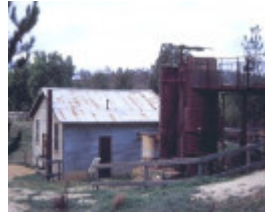
h01322 1 forest creek tourist gold mine castlemaine and chewton road castlemaine engine shed side elevation she project 2003
