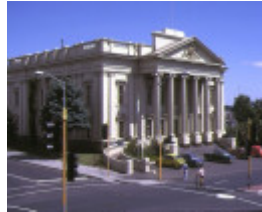
geelong town hall gheringhap street geelong front corner view
