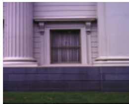
geelong town hall gheringhap street geelong window detail
