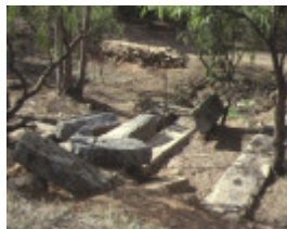
1 golconda glasgow reef golden gully boiler footings may1993
