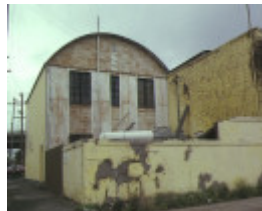
former brown bros iron store mercer street geelong rear view
