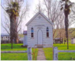
52861 ST. CATHERINE'S ANGLICAN CHURCH (FORMER)
