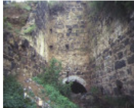
lime kiln complex limeburners point geelong east brickwork detail july 1984
