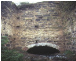
lime4 kiln complex limeburners point geelong kiln detail
