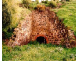
lime kiln complex limeburners point geelong front view
