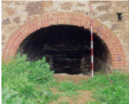
lime kiln complex limeburners point geelong arched entrance publication
