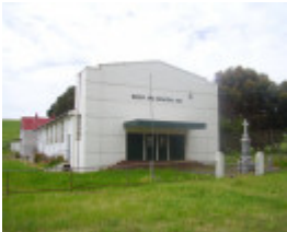
52918 Wando Vale Memorial Hall
