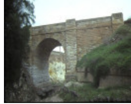
1 bridge over djerriwarrh creek bacchus marsh front elevation sep1984
