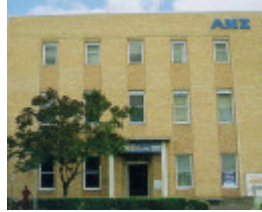
anz bank malop street geelong front elevation publication
