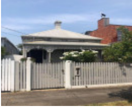
16 Chandlers Road, Malvern
