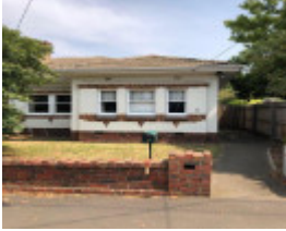
24 Claremont Avenue, Malvern
