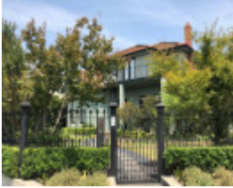
34 Claremont Avenue, Malvern
