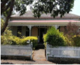
37 Claremont Avenue, Malvern
