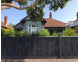
40 Claremont Avenue, Malvern
