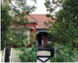
41 Claremont Avenue, Malvern
