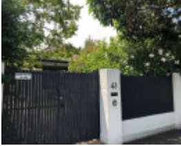
43 Claremont Avenue, Malvern
