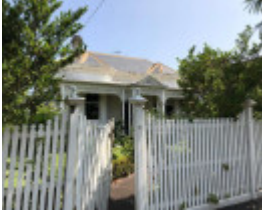
44 Claremont Avenue, Malvern
