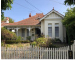
48 Claremont Avenue, Malvern
