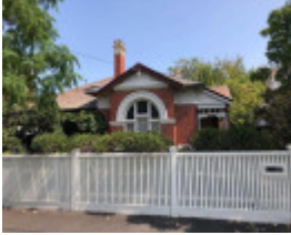
52 Claremont Avenue, Malvern
