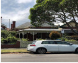
55 Claremont Avenue, Malvern
