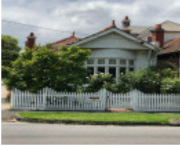
59 Claremont Avenue, Malvern
