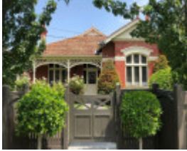
66 Claremont Avenue, Malvern
