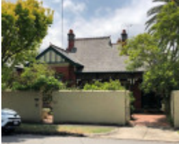
69 Claremont Avenue, Malvern
