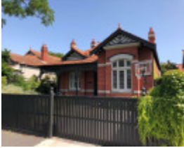
74 Claremont Avenue, Malvern
