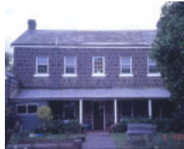
h01387 timboon house old geelong road camperdown back of house she project 2003
