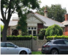
77 Claremont Avenue, Malvern
