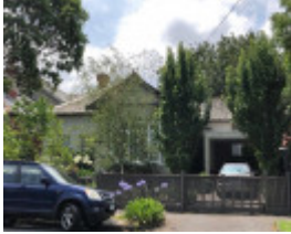
79 Claremont Avenue, Malvern
