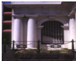
trustees chambers malop street geelong iron work
