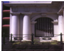
trustees chambers malop street geelong iron work
