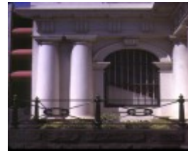
trustees chambers malop street geelong iron work
