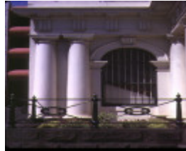
trustees chambers malop street geelong iron work
