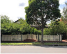
87 Claremont Avenue, Malvern
