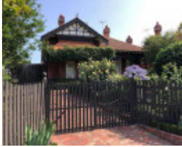
88 Claremont Avenue, Malvern
