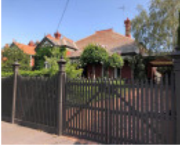
90 Claremont Avenue, Malvern
