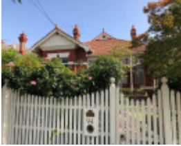
94 Claremont Avenue, Malvern
