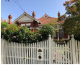
94 Claremont Avenue, Malvern
