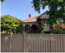
96 Claremont Avenue, Malvern
