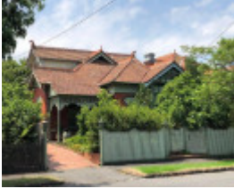
99 Claremont Avenue, Malvern
