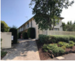
100 Claremont Avenue, Malvern
