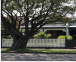
101 Claremont Avenue, Malvern
