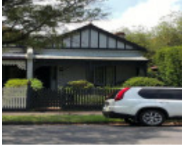
103 Claremont Avenue, Malvern
