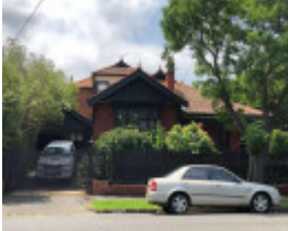
105 Claremont Avenue, Malvern
