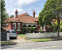
111 Claremont Avenue, Malvern
