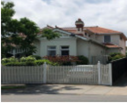
117 Claremont Avenue, Malvern
