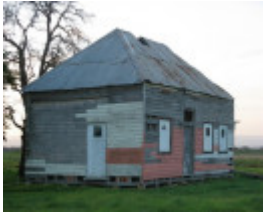
Residence Stawell Street Tarraville small
