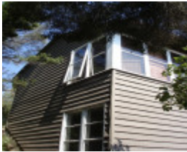
5345 Ramsay House Mt Eliza Enclosed North West Corner 23 March 2006 mz
