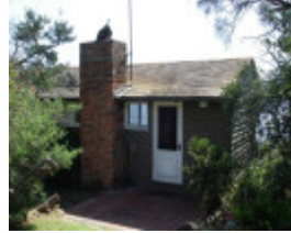
5345 Ramsay House Mt Eliza Enclosed Bedroom Balcony 23 March 2006 mz
