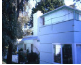
h01910 the ship rannoch ave mt eliza back exterior she project 2003
