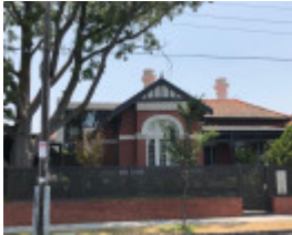
17 McKinley Avenue, Malvern
