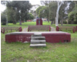
Before Photograph - Reference F3921 2014
