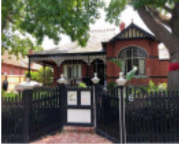
6 Staniland Avenue, Malvern
