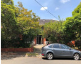
13 Staniland Avenue, Malvern
