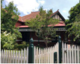
18 Staniland Avenue, Malvern
