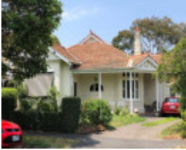
21 Staniland Avenue, Malvern
