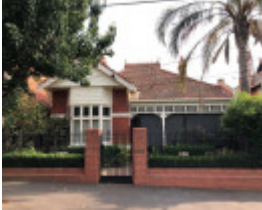
113 Station Street, Malvern
